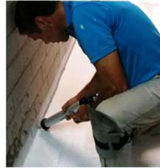
Wet Area Waterproofing
